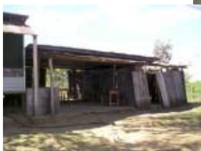
Old extension building
