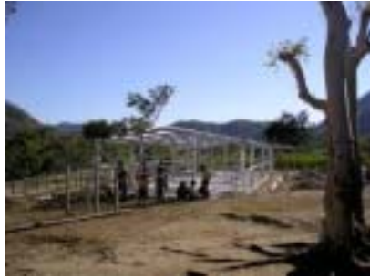
Framework for new building
